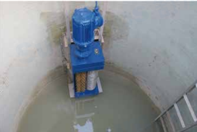
Installation photo of the grinder screen in a prefabricated pump station
