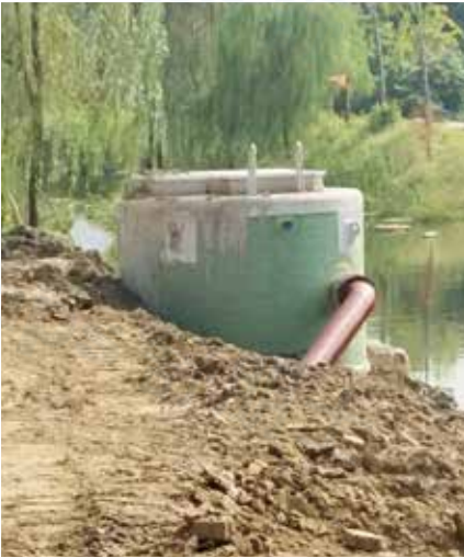
This project remediates 11 existing stormwater outfalls on the Guanhe River, Zhuxi River, and Cooling River. For 6 outfalls with dry-weather sewage discharge, Integrated Smart Interception & Lifting Chambers will be installed; the remaining 5 already intercepted outfalls will undergo intelligent retrofitting.
